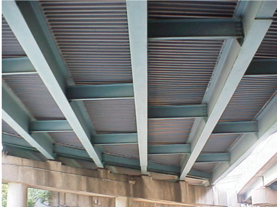
Figure 5.2.1 Stay-in-Place Forms
