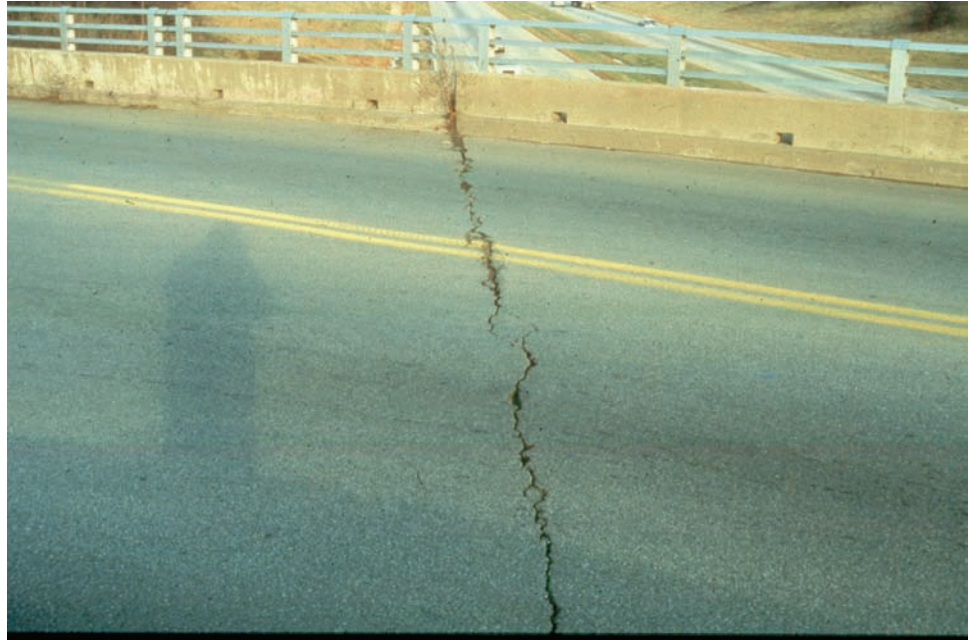
Figure 5.4.19 Asphalt Wearing Surface over an Expansion Joint
