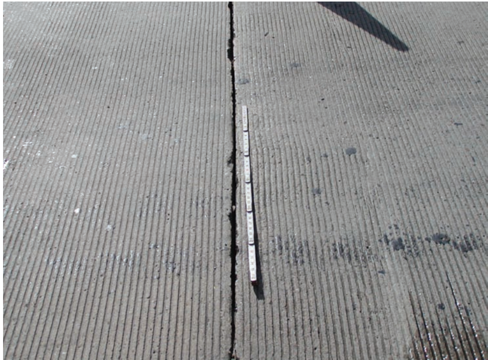
Figure 5.4.1 Formed Joint
