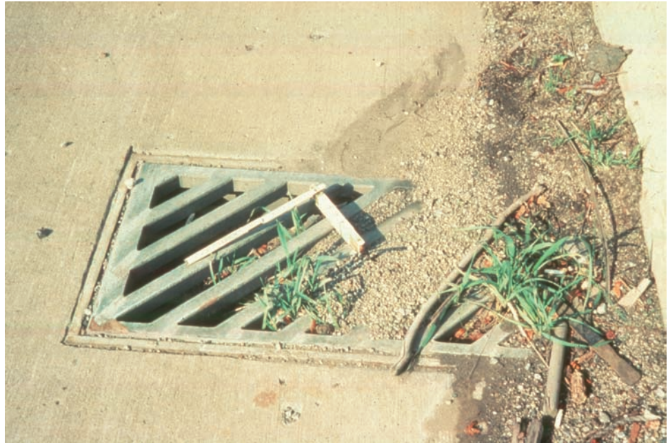
Figure 5.4.13 Bridge Deck Drain
