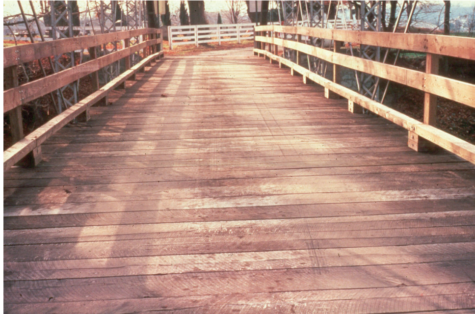
Figure 5.1.1 Plank Deck
