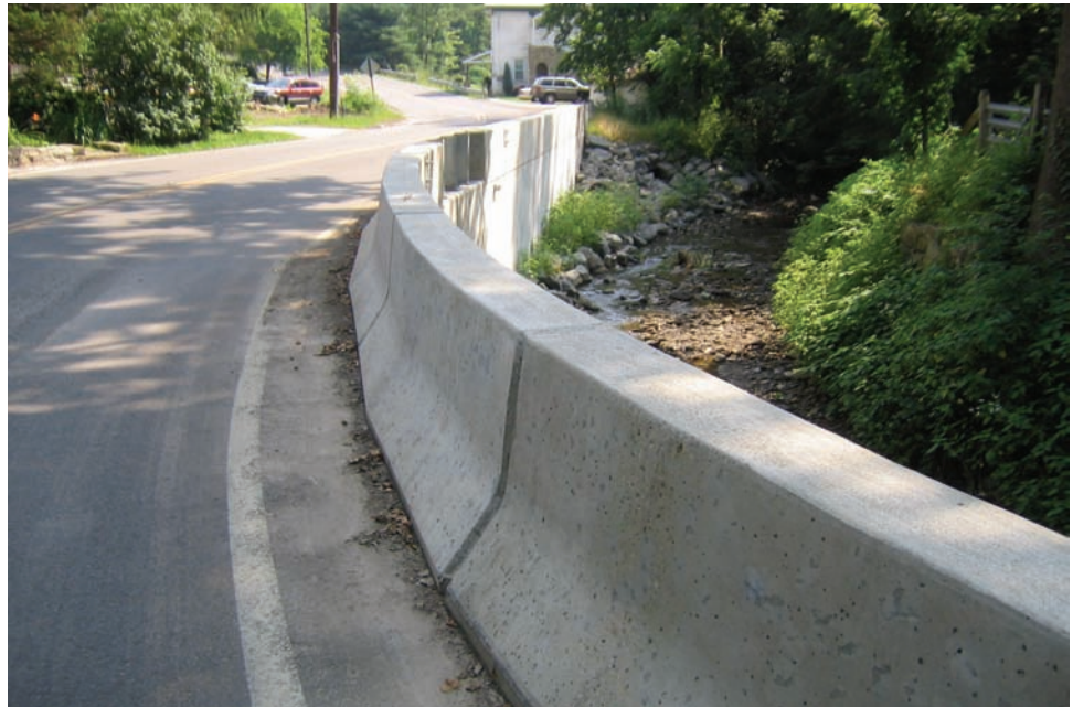
Figure 5.5.4 Acceptable Bridge Rail
