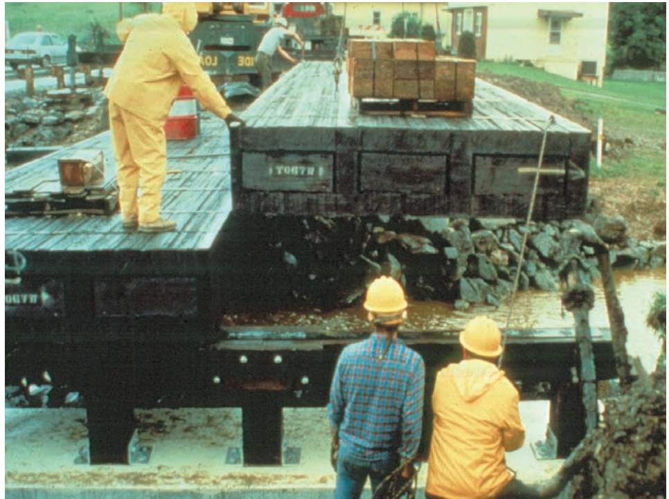
Figure 5.1.5 Structural Composite Lumber Deck Using Box Sections
