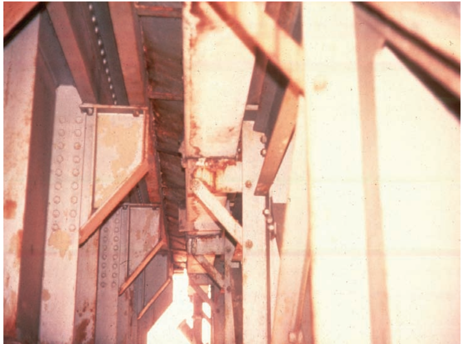
Figure 5.4.5 Supported Finger Plate Joint
