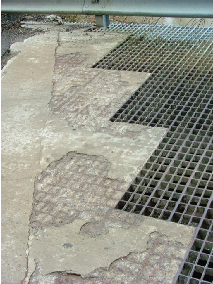
Figure 5.3.5 Filled and Un-filled Steel Grid Deck
