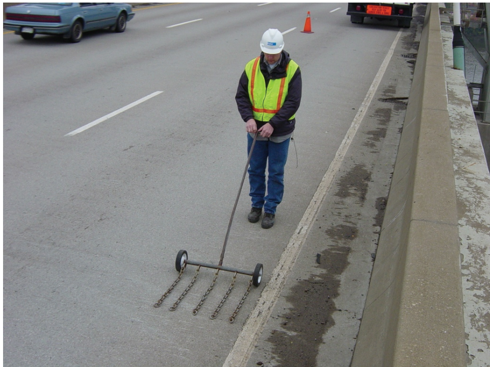
Figure 5.2.10 Sounding for Delaminated Areas of Concrete
