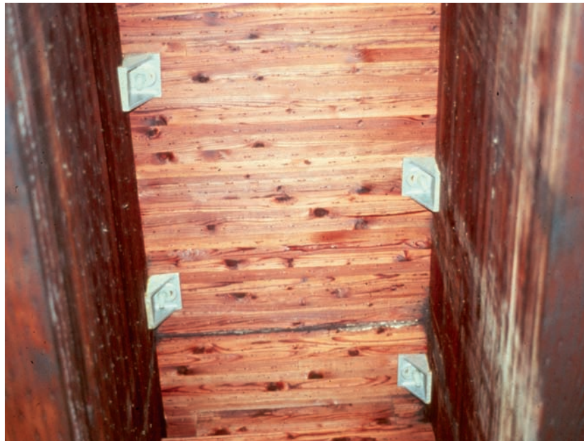
Figure 5.1.3 Glued-laminated Deck Panels
