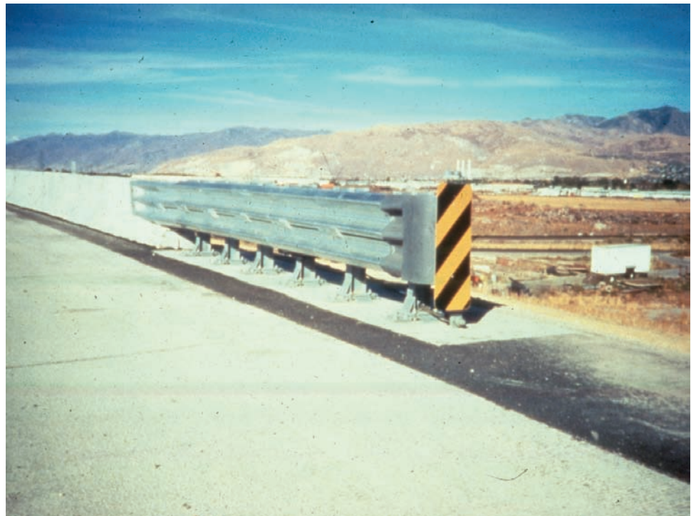
Figure 5.5.1 Bridge Safety Feature
