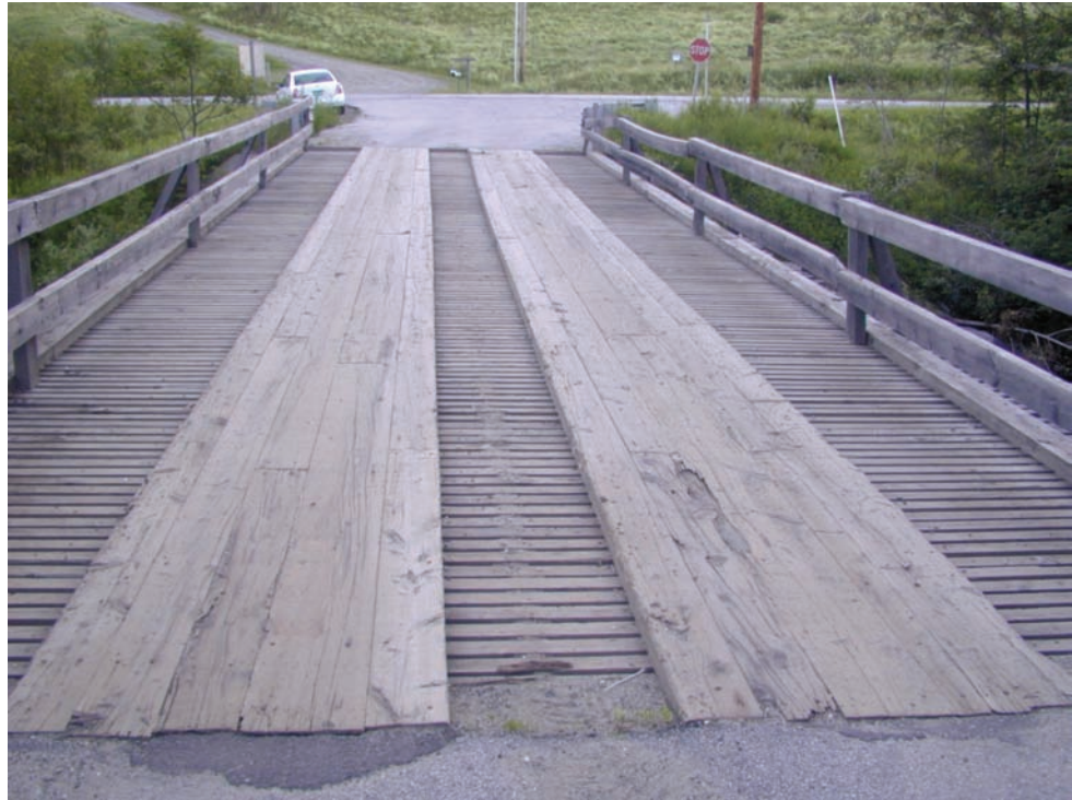
Figure 5.1.6 Timber Wearing Surface on a Timber Deck
