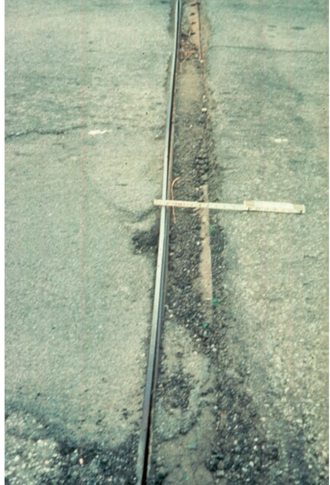
Figure 5.4.15 Debris Lodged in a Sliding Plate Joint
