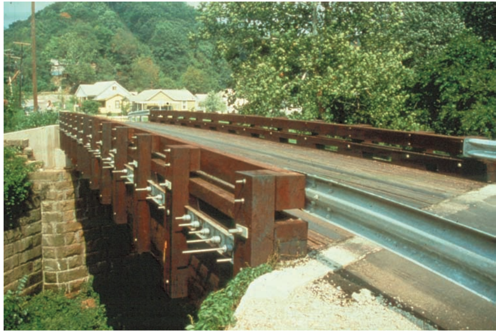
Figure 5.1.4 Stressed-laminated Deck
